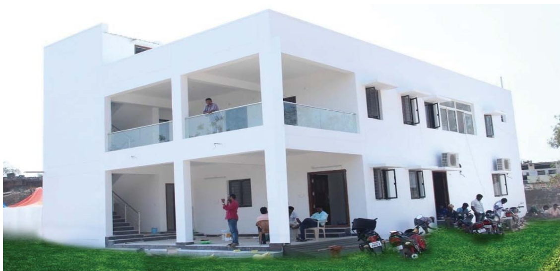
MLA Office- cum -Residence, Parkal
