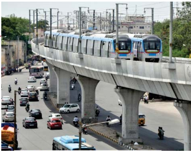
Metro Rail elevated viaduct – with two trains
