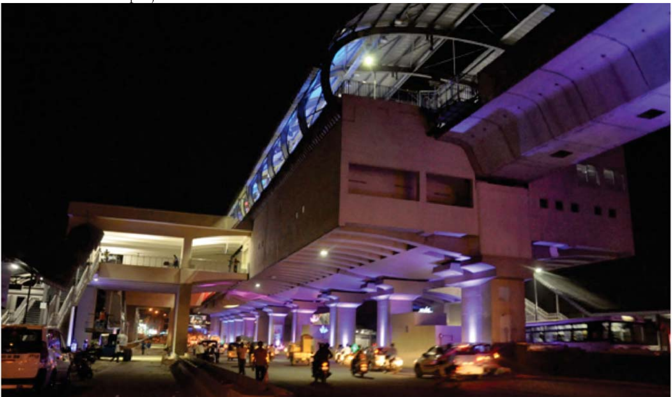
Hyderabad Metro Rail Project
