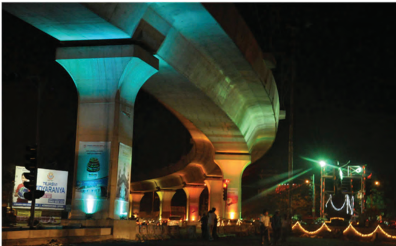
Hyderabad Metro Rail Project
