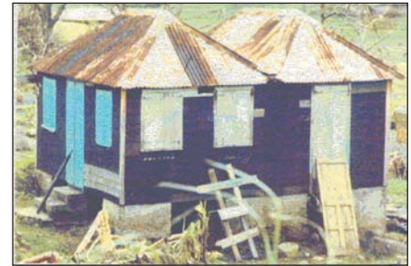
Fig 1. If natural elevation is not available construction on stilts or on artificially raised earth mounds
