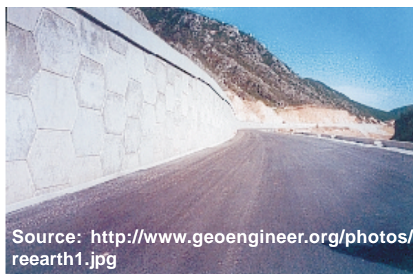
Fig. 2.6.7 Retaining wall - Reinforced wall constructed as a mitigation measure.
