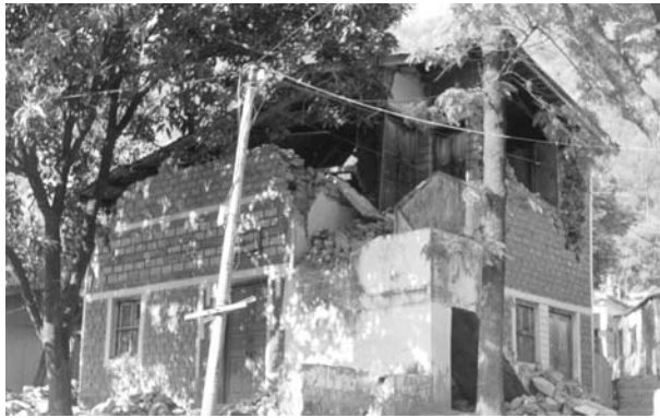
Figure 7.1 : A Damaged Building Due to an Earthquake
